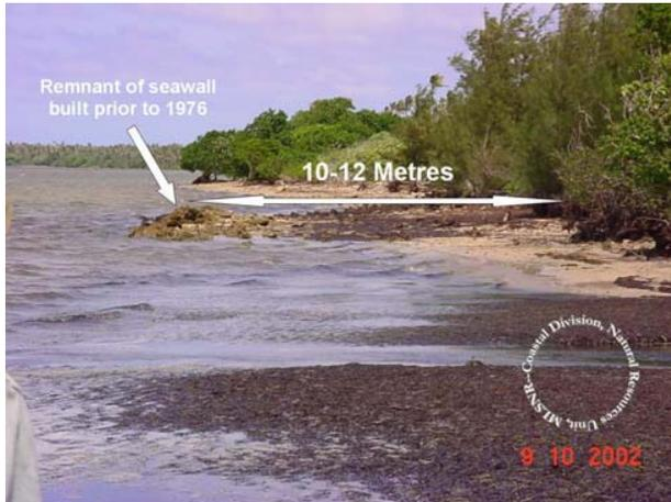
Landward migration of the shoreline is also presumed from fieldwork observations, indicated by fallen trees and exposed tree roots on the shoreline. Remains of possibly an old protection seawall built before 1976 stands 10 - 12meters seaward from the present shoreline also indicate recession of the land (Plate 4.8).
