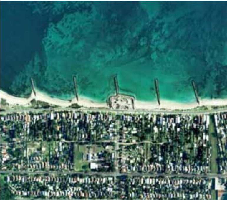
Figure 45: Groynes at Botany Bay, New South Wales, Australia
