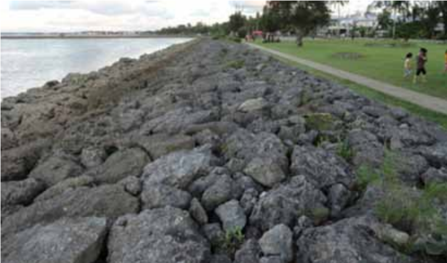
Figure 37: Rock revetment, Nuku'alofa
