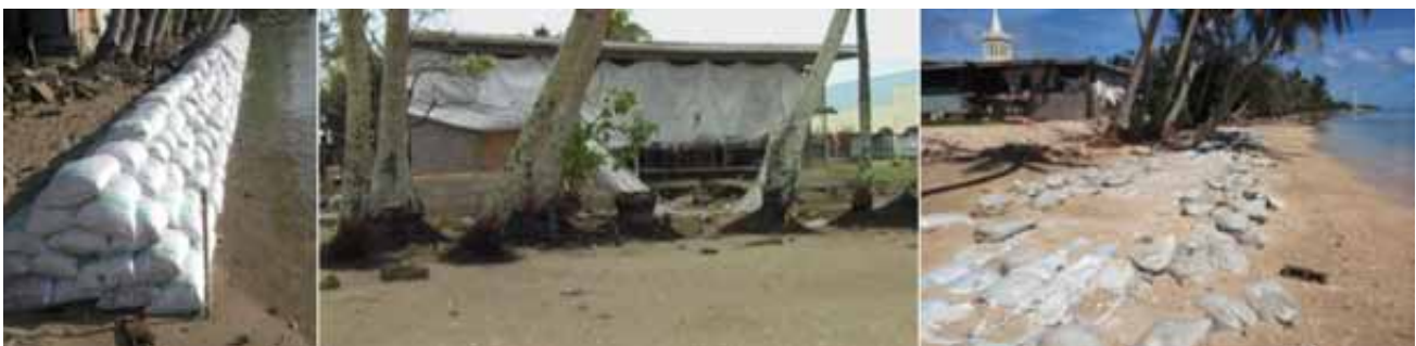
Figure 5: A sea wall project in Hihifo before, during and after Tropical Cyclone Rene (2010)
