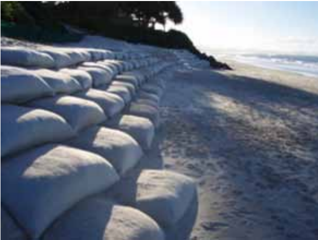
Figure 40: Sand-filled geotextile container revetment at Byron Bay, New South Wales, Australia
