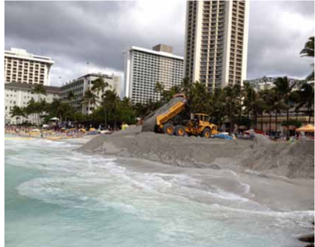
Figure 43: Beach recharge work in progress
