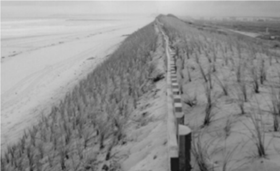
Figure 49: Beach nourishment project at Jimmy's Beach, Port Stephens, New South Wales, Australia
