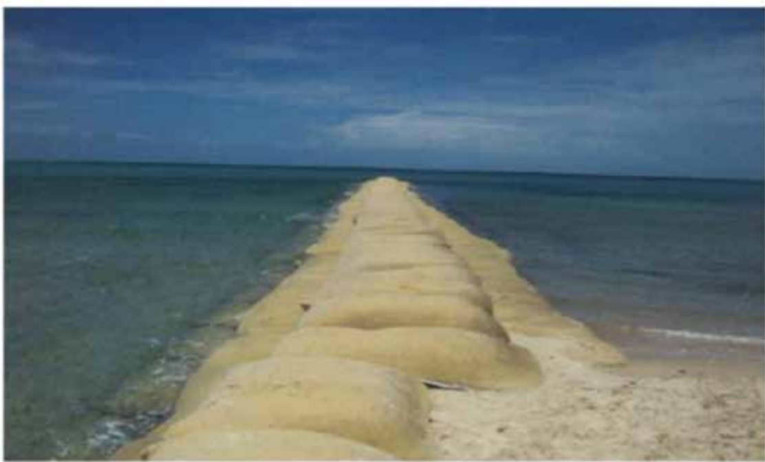
Figure 46: Groyne made of geotextile bags
