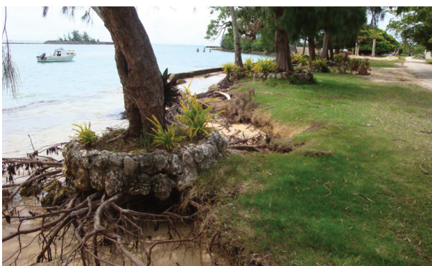
FIGURE 3-44 Erosion at lifuka
