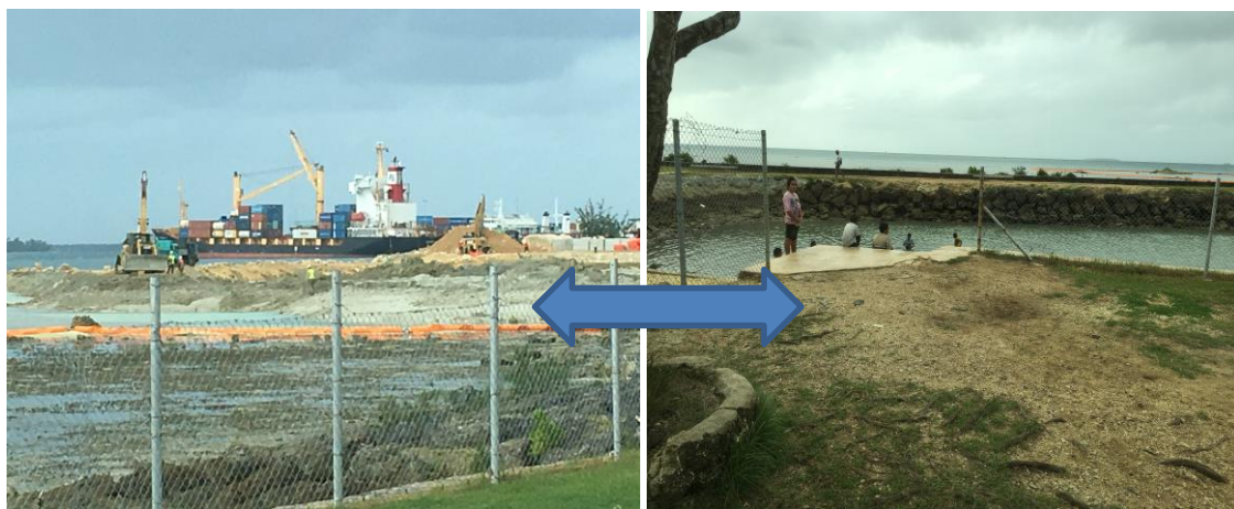
Figure 9: Construction of the Wharf
