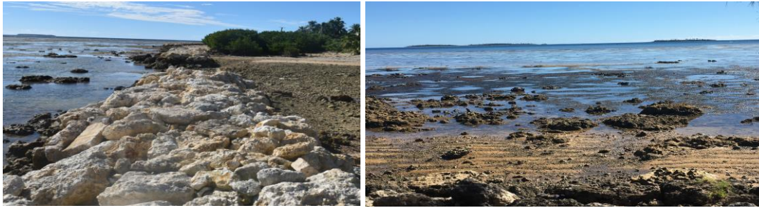
Figure 10: Fore shore construction
