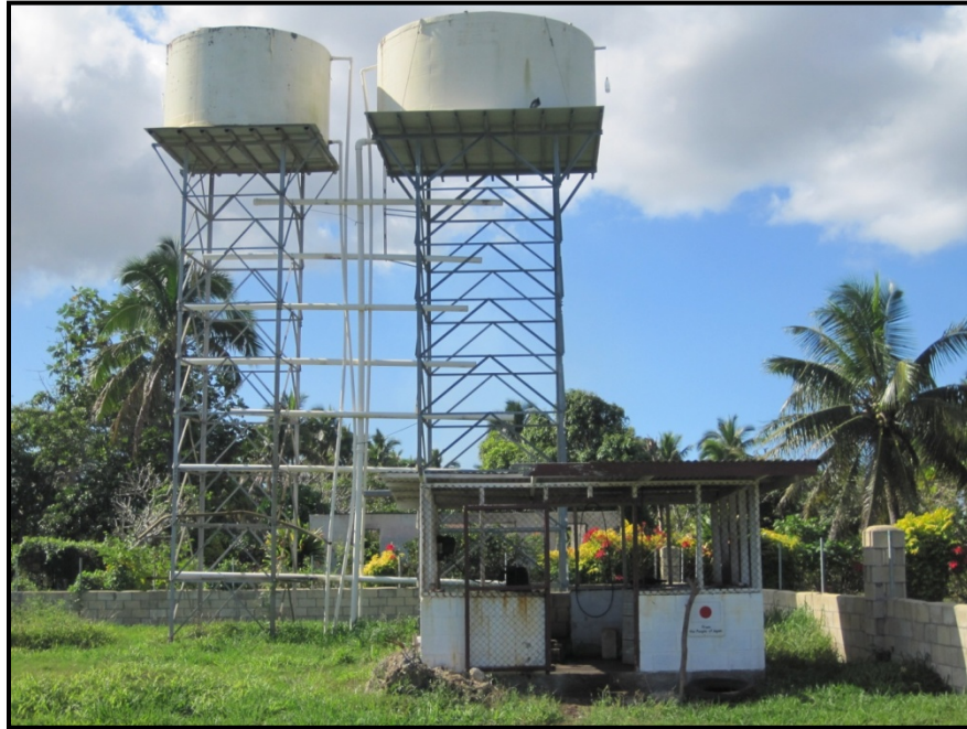
Figure 13: 'Utulau village well supply (Tongatapu), showing pump house and reservoir. (Nicola Fry, 2010)
